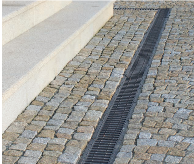
4-25 Outdoor drains Due to its unique characteristics it offers maximum variability as well as good load capacity and durability.
